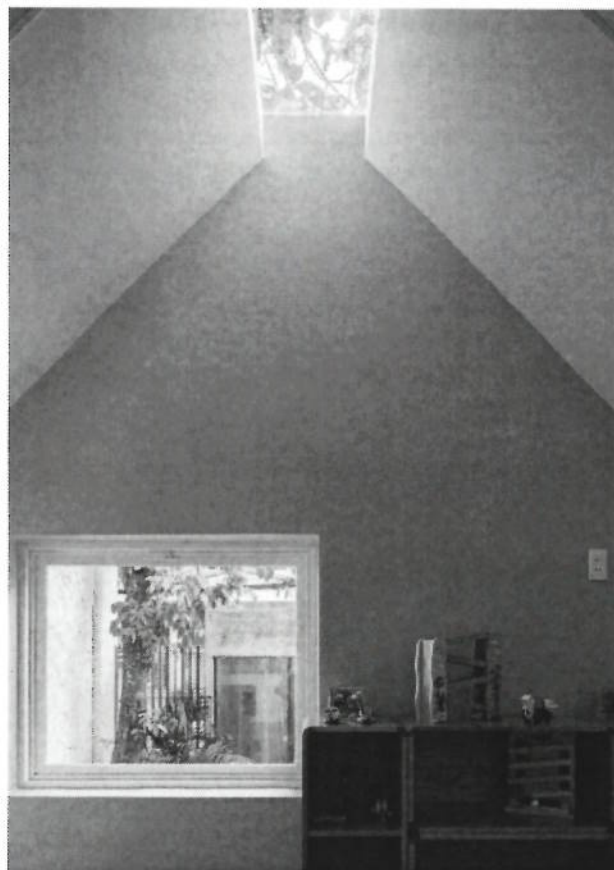
Figure 2-9 Skylights can help improve natural light into activity rooms.
